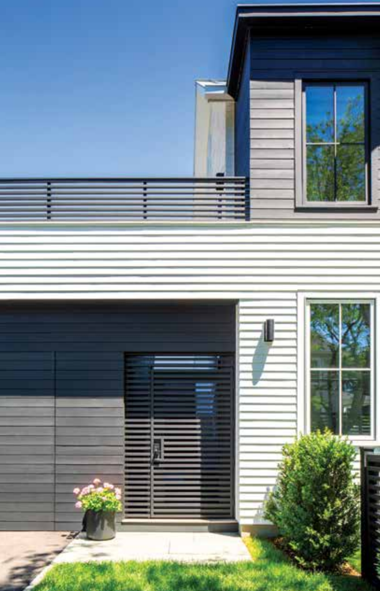
LEFT: The exterior features a mix of white clapboard siding and stained western red cedar siding and railings; a door between the house and garage conceals an open-air staircase leading to the balcony above the garage. BELOW: The living and dining areas and the kitchen are open to one another, but clutter is kept at bay. “We didn’t want people putting their coats on the back of the sofa when they walked in,” says the homeowner. “An idea that started as a screen, which felt cold and one-dimensional, ended up as a bookshelf. It brings the entire space together.”
